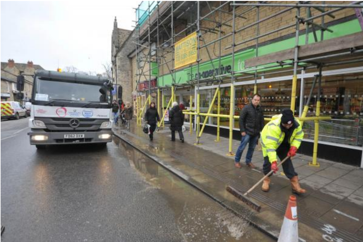
Flooding: Cleaning up Witney High Street
